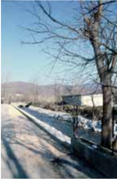
A straightened and cemented stream stretch which has completely lost its natural aspect
