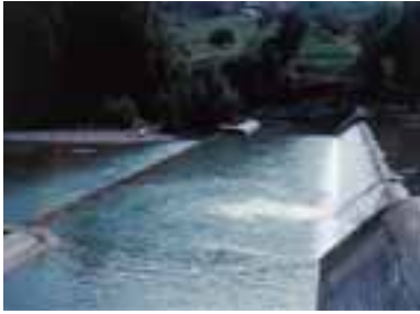
Embankment and preventer bobstay in the river Panaro (Emilia)
