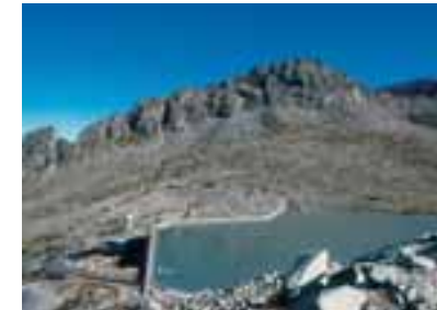
Artificial lake of Venerocolo (Adamello) exploits a lateral moraine as a bank
