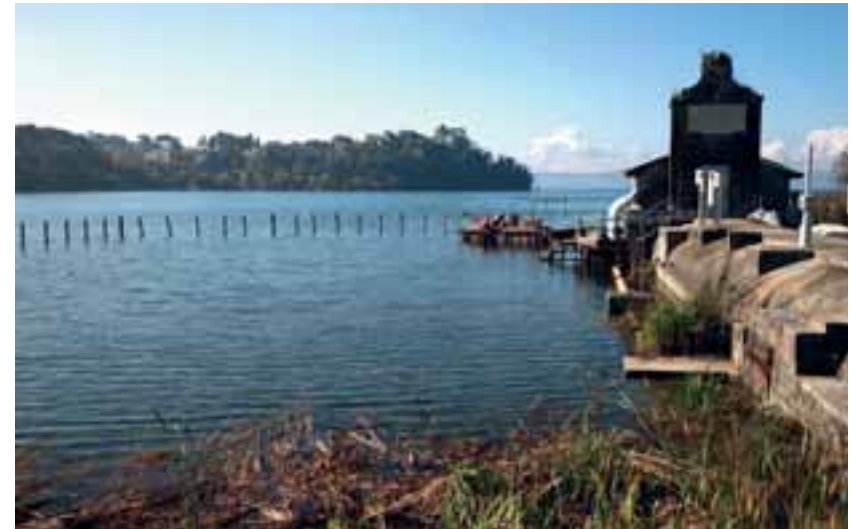
Water pumping station on Lake Bracciano (Latium)
