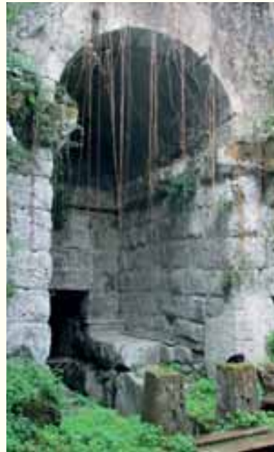
The artificial outlet built by the Romans in 394 BC to regulate the level of Lake Albano
