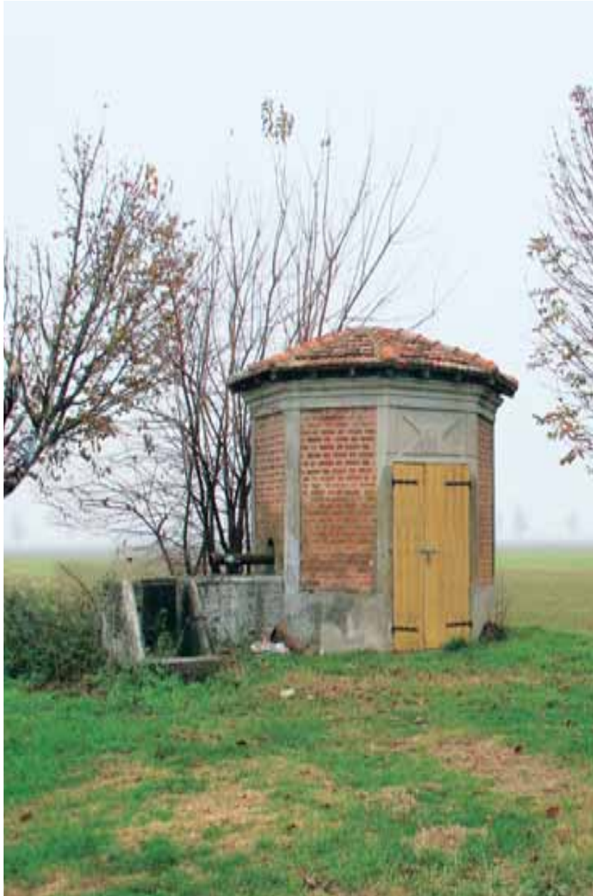
An old "pumping-house" (Viarolo, Emilia Romagna)
