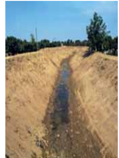
Construction of a diversion channel
