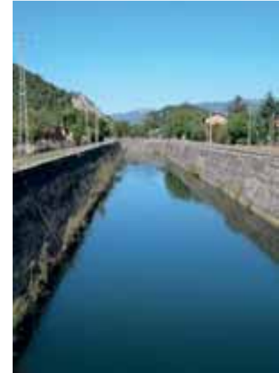
Canal for hydroelectric purposes (Umbria)
